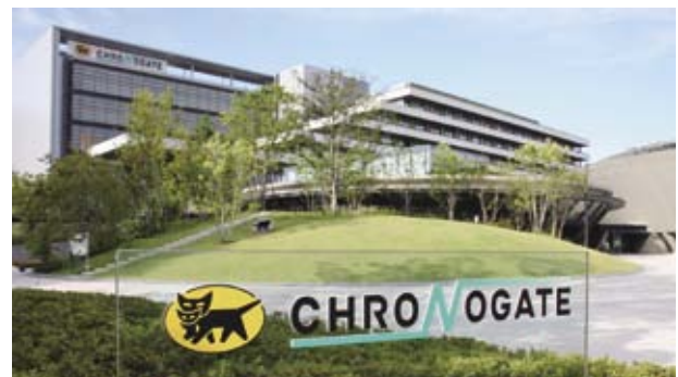
Realizing high efficiency and cost reduction by introducing the inspection support system into the YSD warehouse located in "Haneda Chronogate," Yamato group's total logistics terminal, and contributing to our comfortable lifeline.
